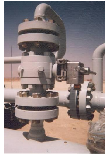
Ball valve with an Interlock installed
